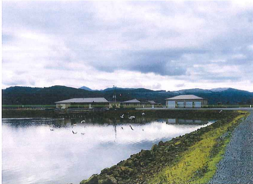
Treatment Plant near Lagoon A
